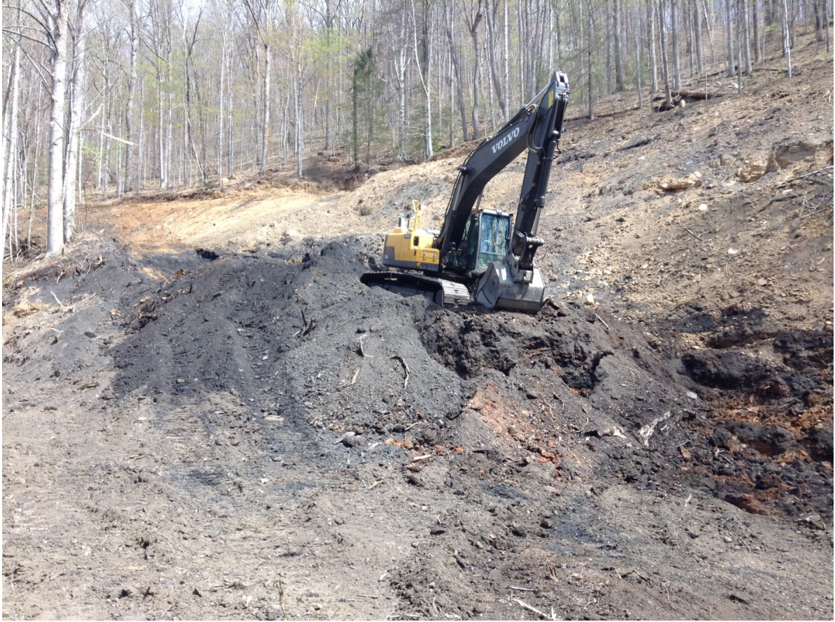
Figure 3. Coal refuse extraction at the Cove Creek site on 4/21/2014.
