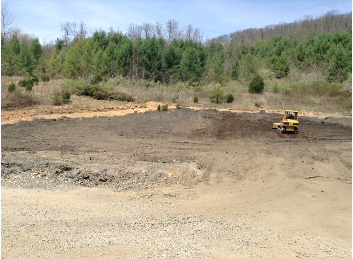
Figure 4. Extracted coal refuse being spread out at the disposal site on 4/21/2014.
